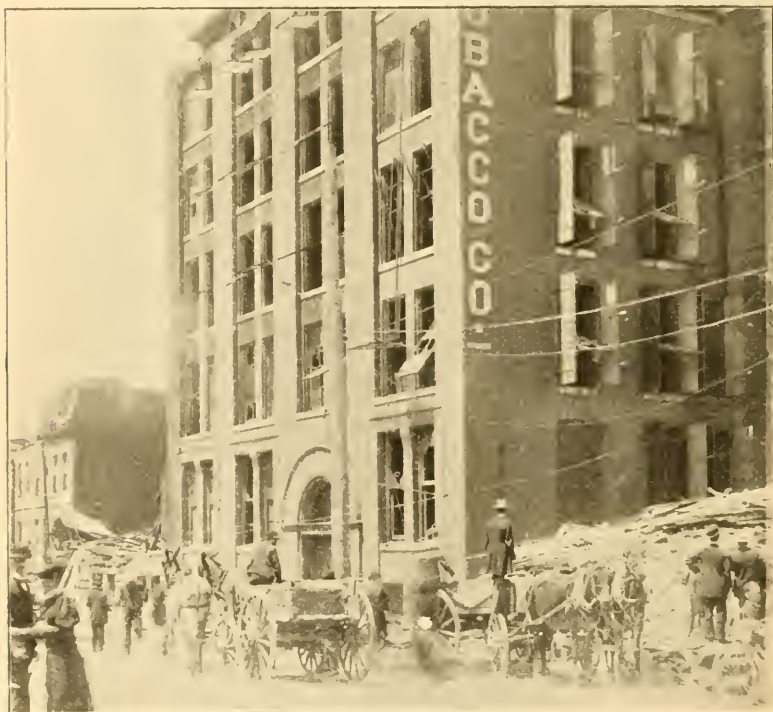
BROWN TOBACCO COMPANY'S BUILDING. (FOUR PERSONS WERE KILLED IN THE WRECK ON THE RIGHT.)
